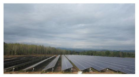
The solar plants are expected to generate 9,4000 MWh of electricity per year, enough to power approximately 24,000 households, while reducina approximately 56,000 tons of carbon emissions and 30,174 tons of fossil fuels annually.
