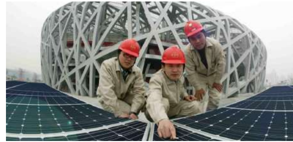
Beijing National Stadium BIPV Project
