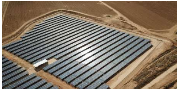
Enlight Kramim PV Plant
