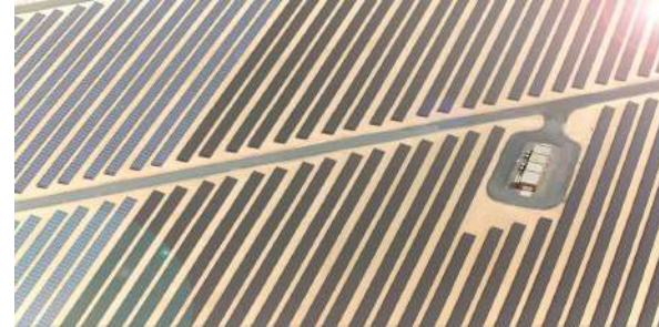
Masdar PV Plant
