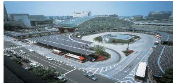
Kanazawa Bus Station BIPV Project
