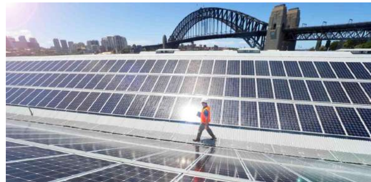
Sydney Opera House Rooftop PV Project
