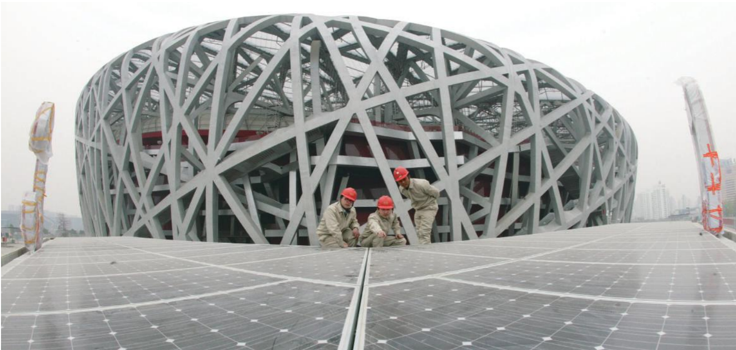
Beijing Bird's Nest Stadium BIPV Project
